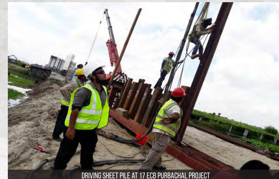
DRIVING SHEET PILE AT 17 ECB PURBACHAL PROJECT
