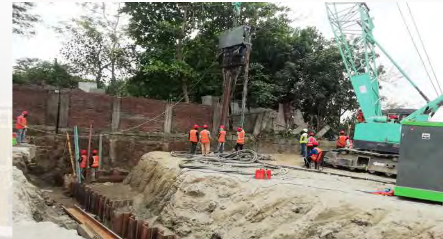
DRIVING SHEET PILE AT HEIDELBERGCEMENT BANGLADESH LIMITED, KANCHPUR, NARAYANGANJ
