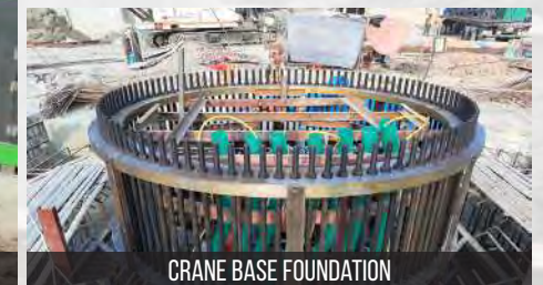
CRANE BASE FOUNDATION
